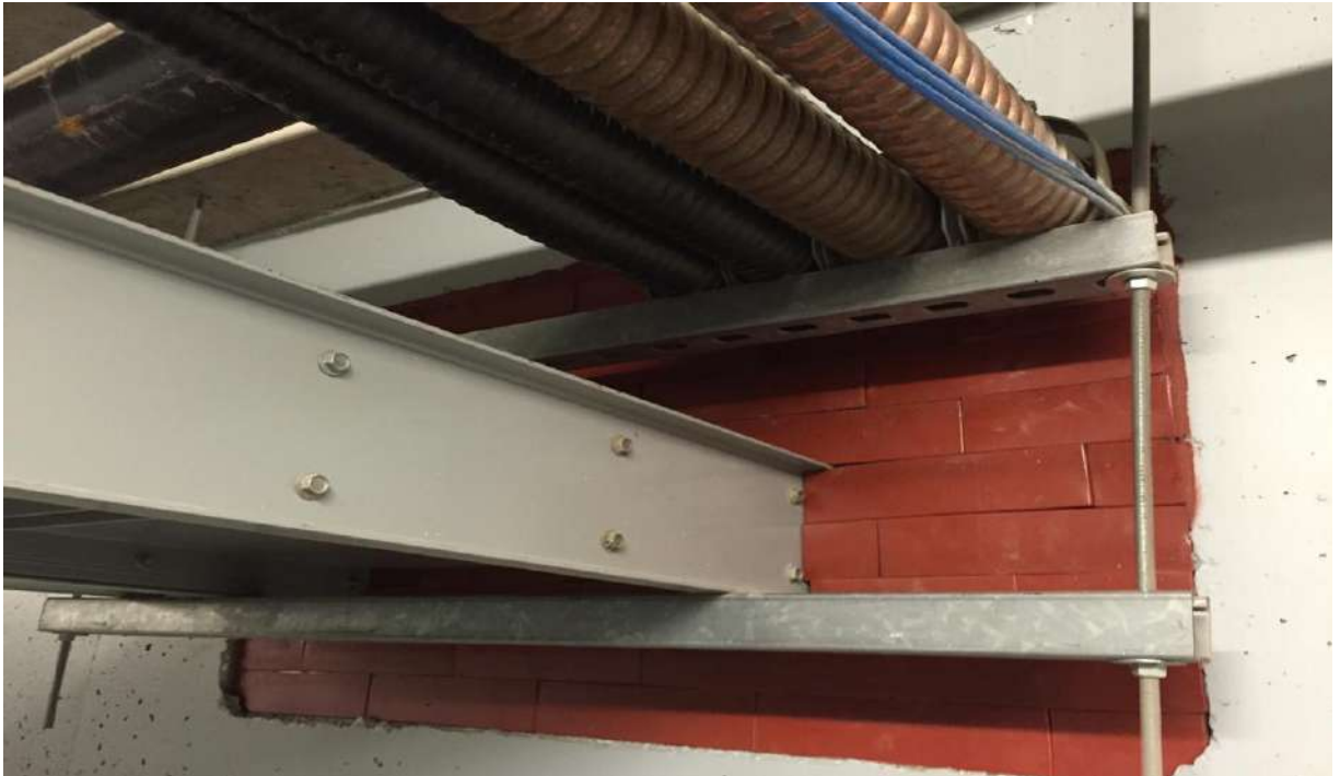
Firestop Bricks for Large Openings
