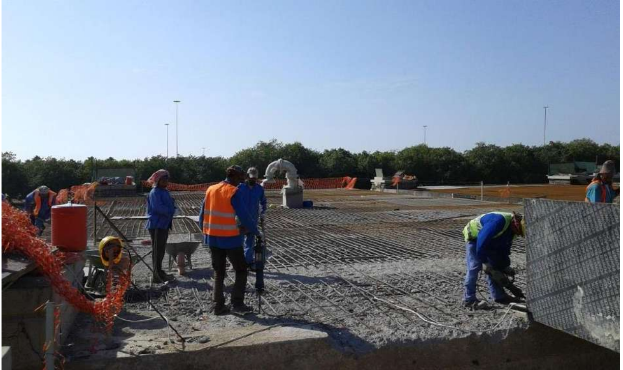
Repair of Concrete Slab
