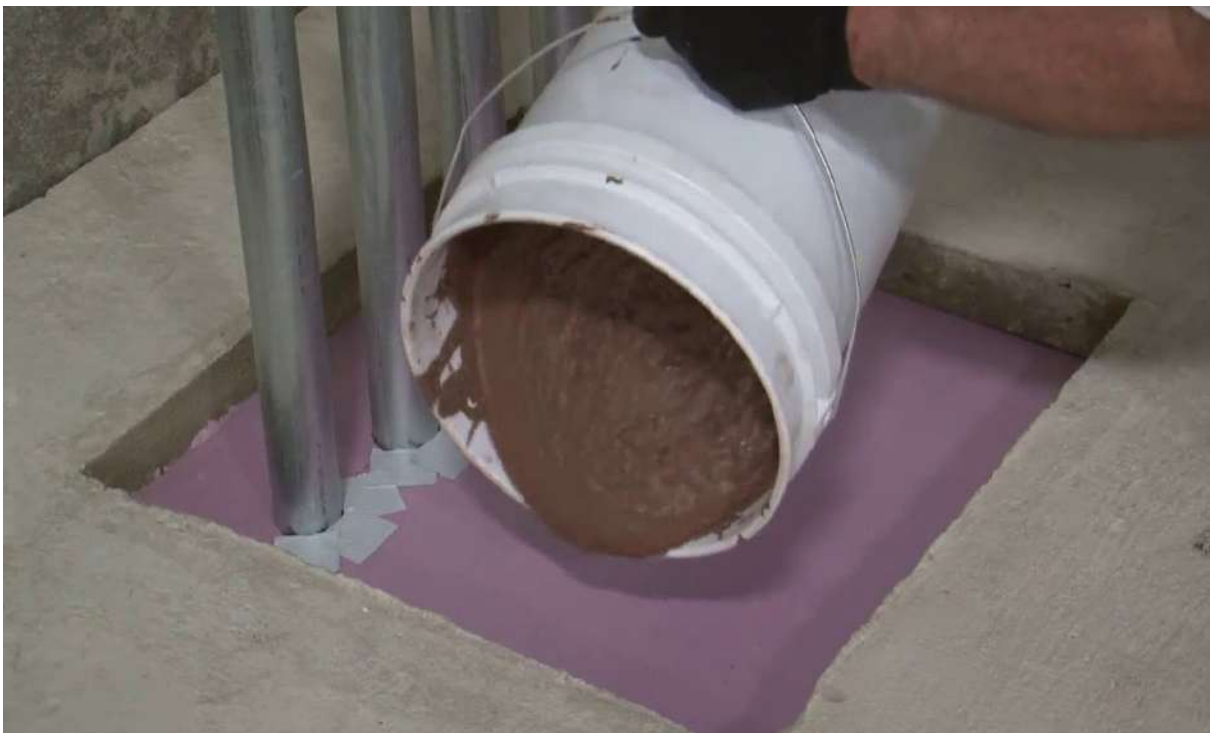
Firestop Mortar for Large Openings
