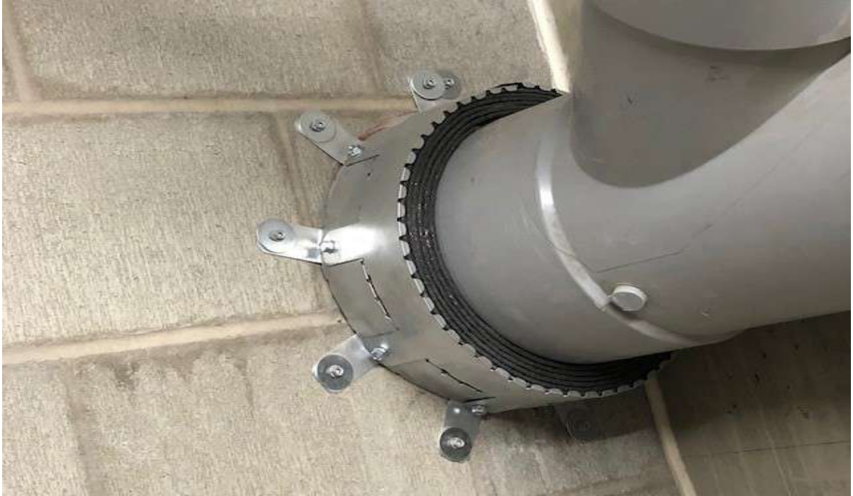
Pipe Thru-Penetration – Intumescent Firestop Collar
