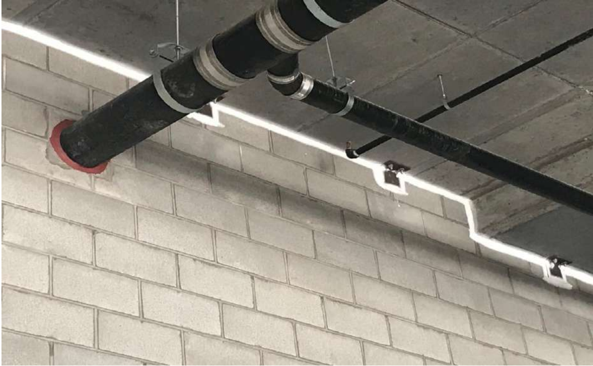
Linear Joint – Sealant Application
