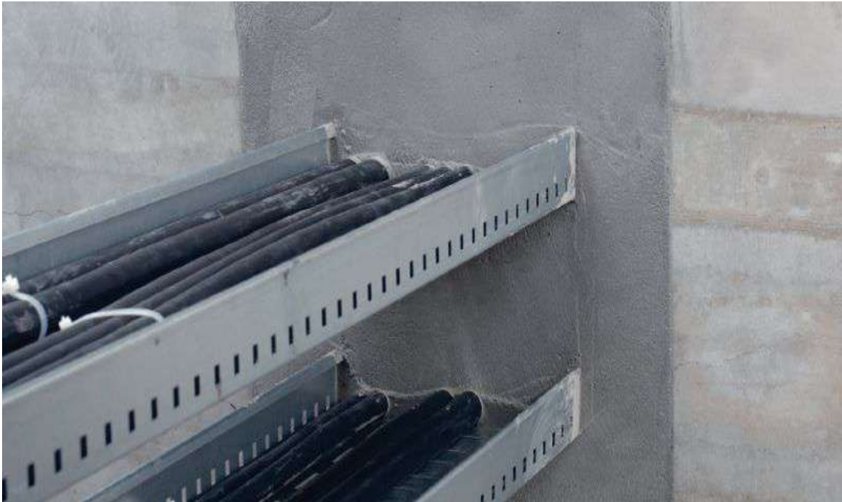
Firestop Mortar for Large Openings
