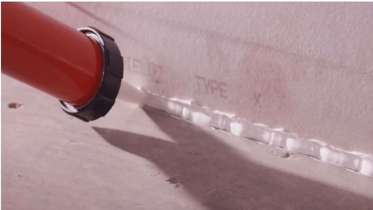
Bottom Of Wall Joint – Sealant Application
