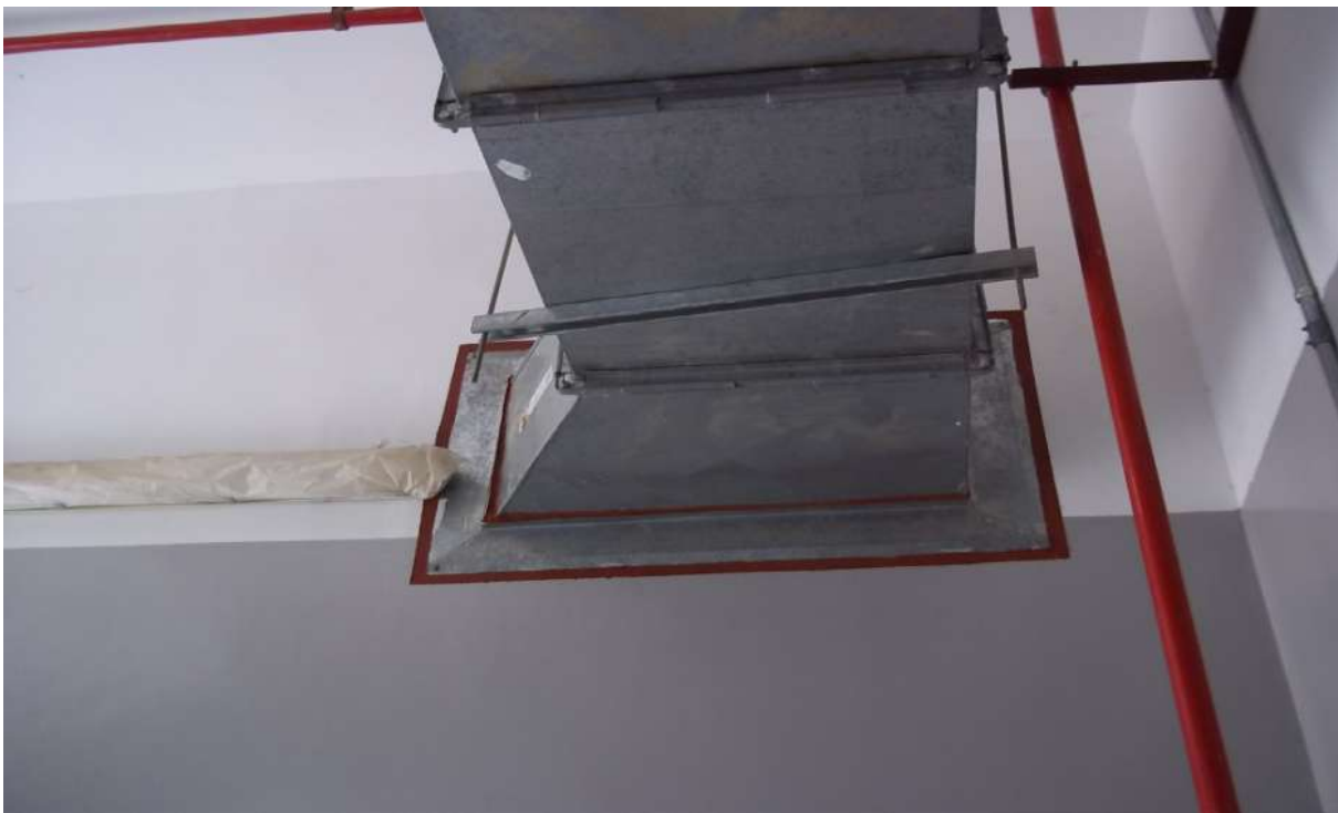
HVAC Ducts – Firestop Sealant
