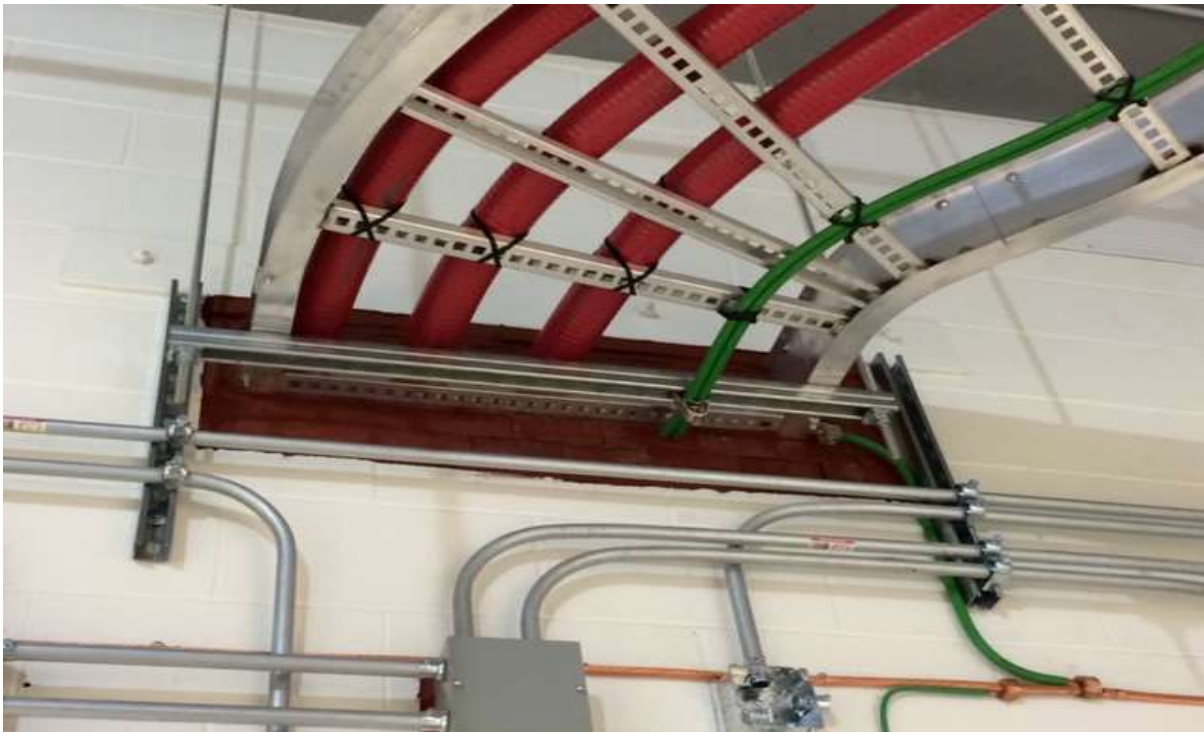
Cable Tray Penetration
