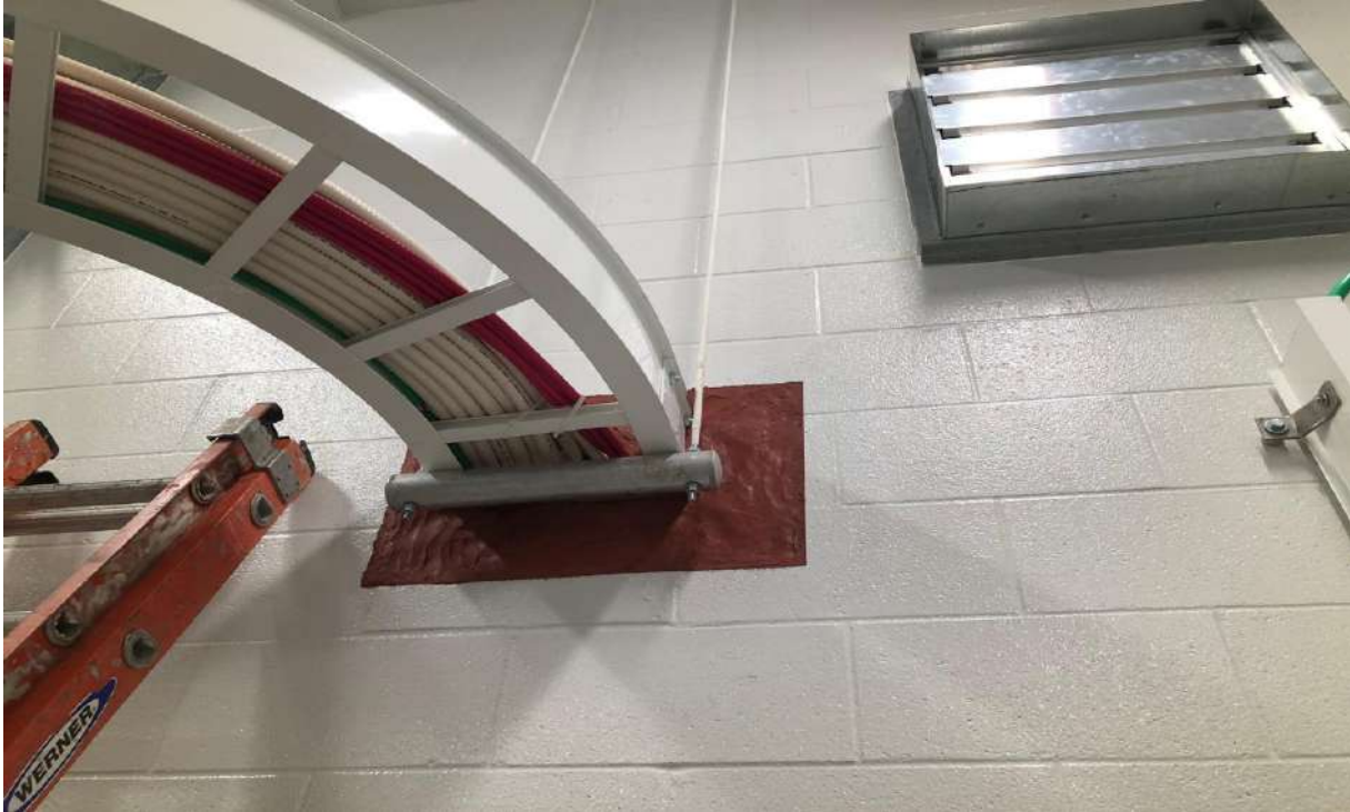
Cable Tray Penetration
