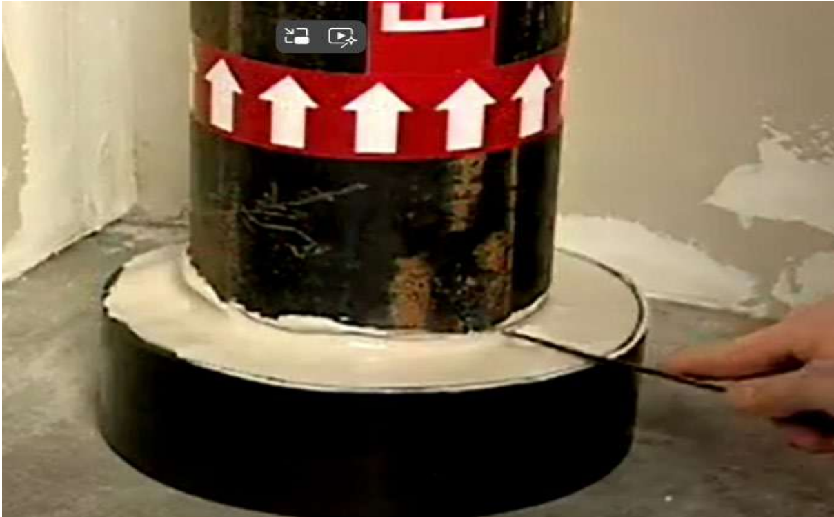
MEP Penetrations – Firestop Mortar
