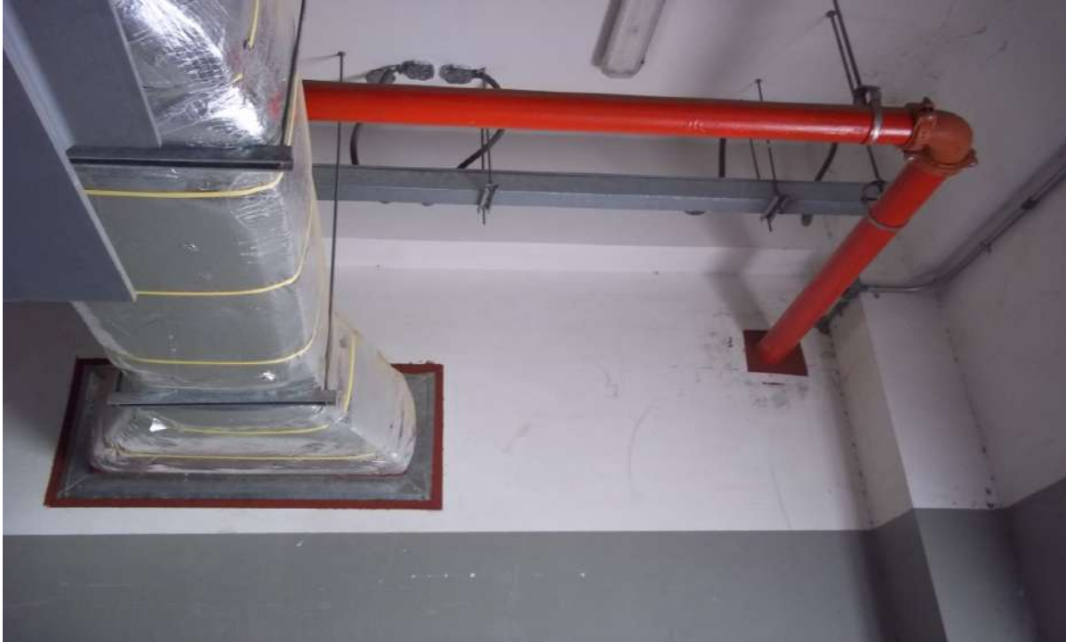
HVAC Ducts – Firestop Sealant
