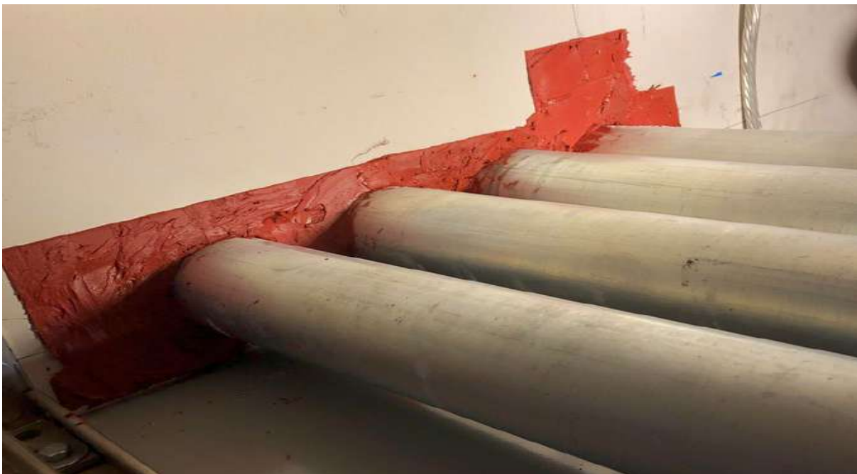
Multiple Penetration - Sealant Application
