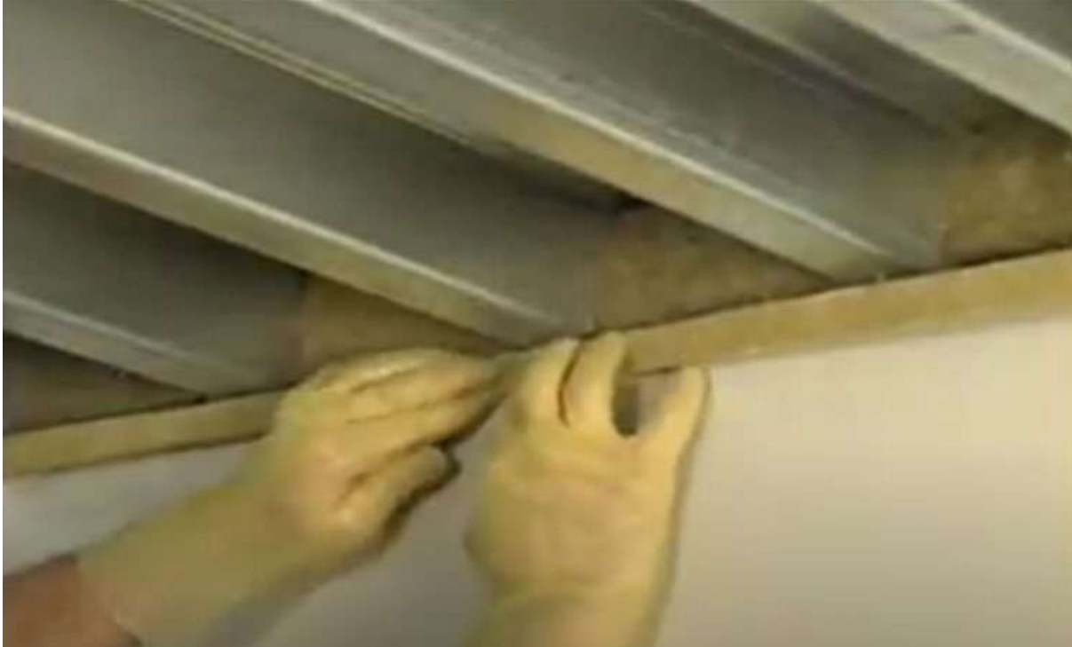
Installation of Rockwool
