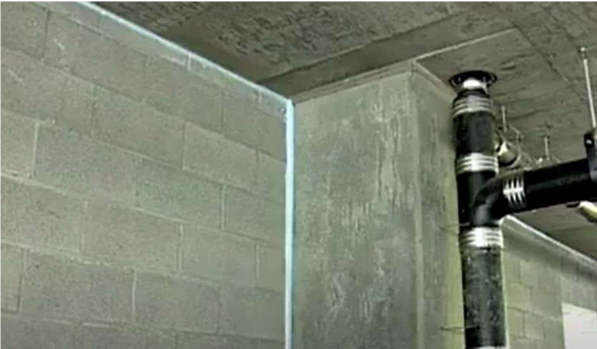
Joint – Sealant Application
