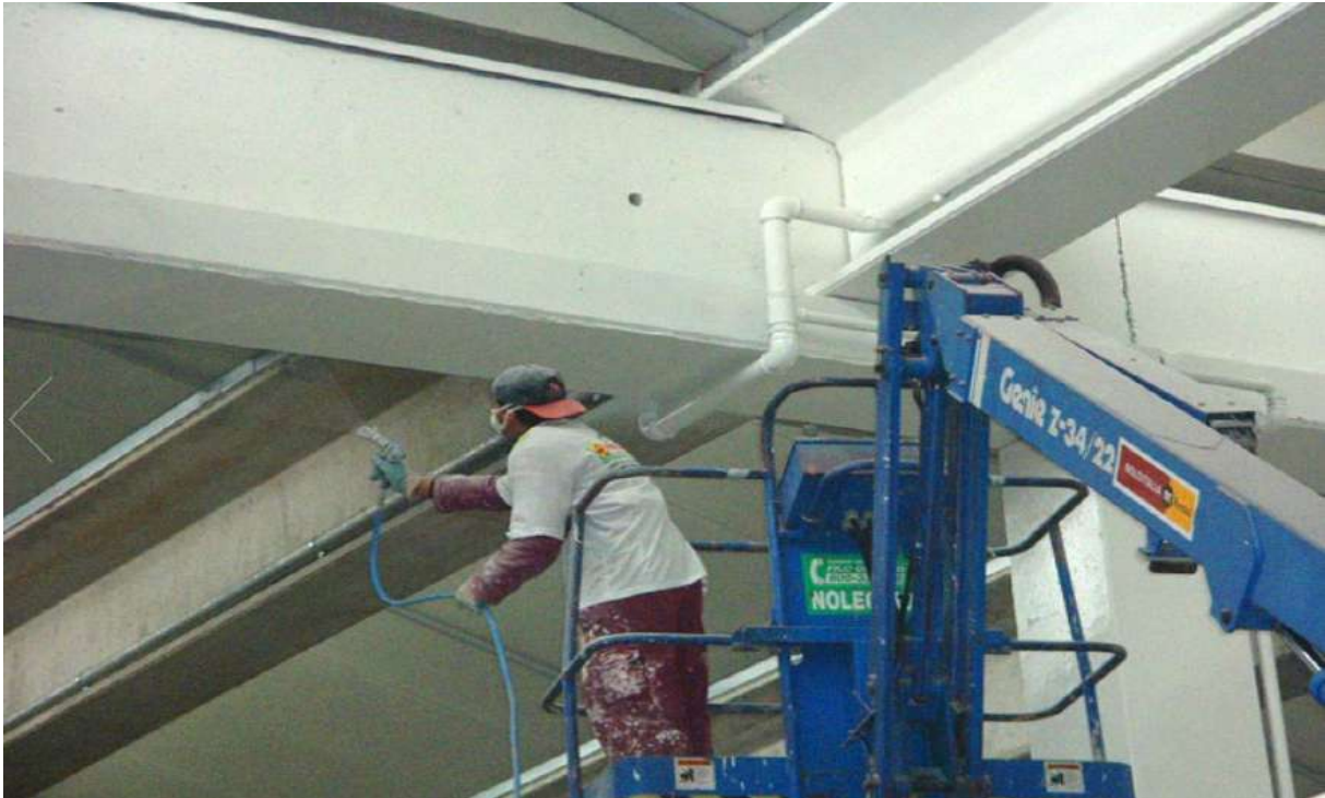
Intumescent Firestop Coating for Steel Structures
