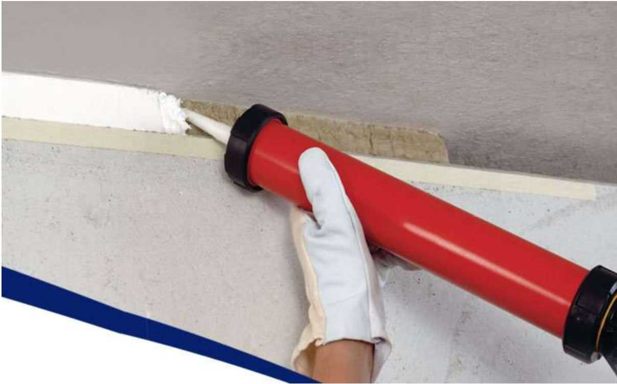
Top Of Wall Joint – Sealant Application
