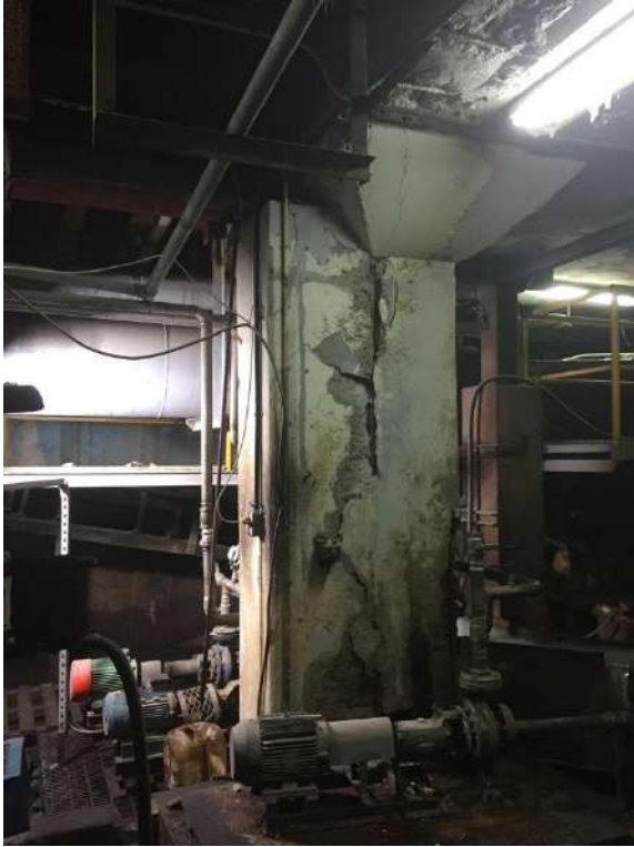
Before Repair Of Column
