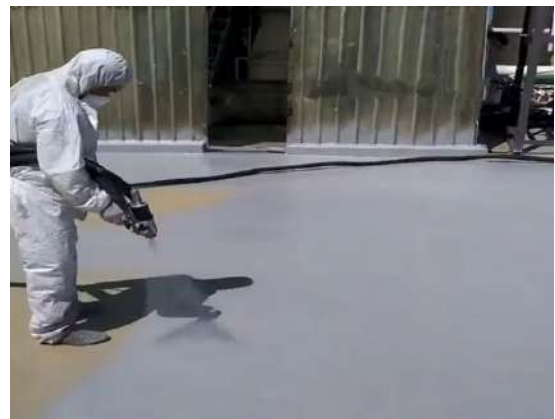
Application of Polyurea Coating
