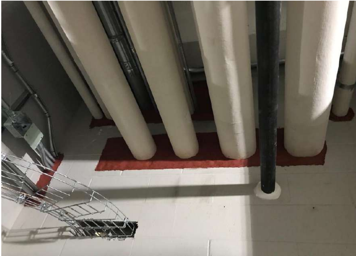
Multiple Penetration - Sealant Application
