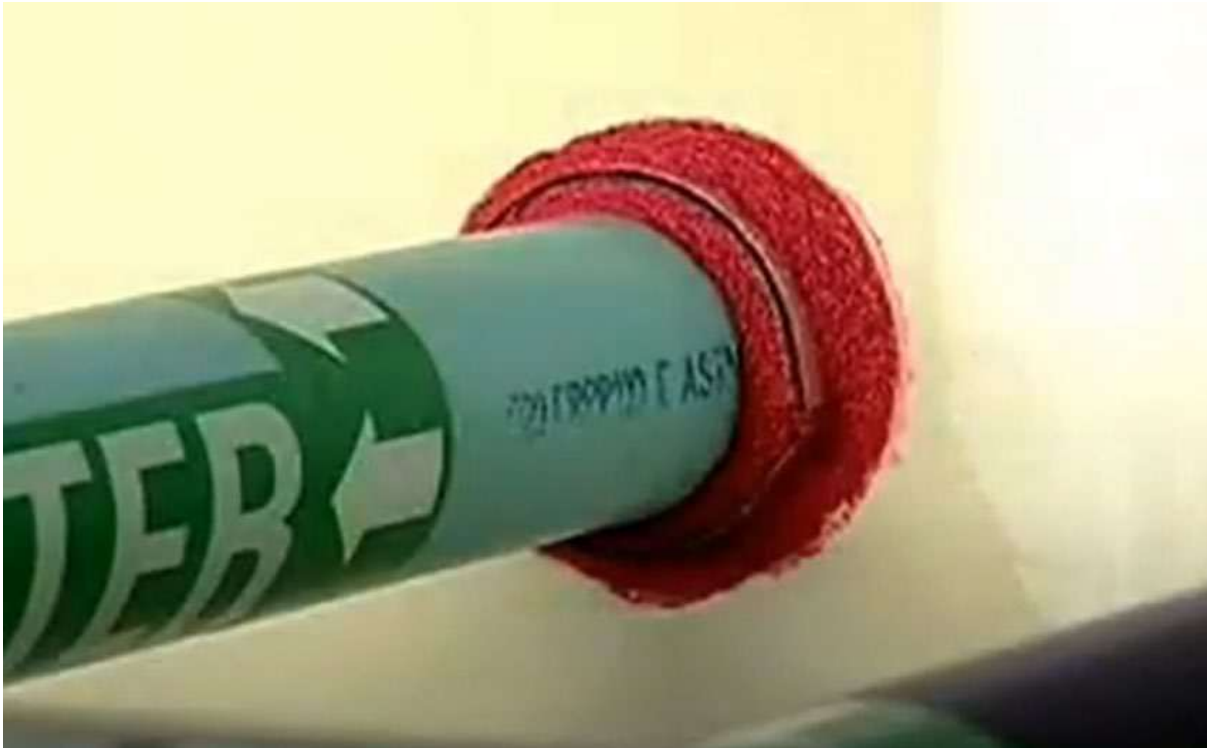
Pipe Thru-Penetration - Intumescent Sealant Application
