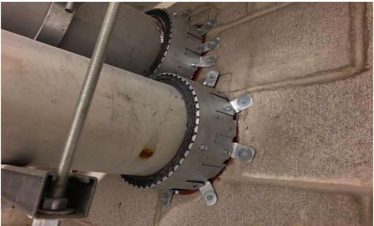
Pipe Thru-Penetration – Intumescent Firestop Collars
