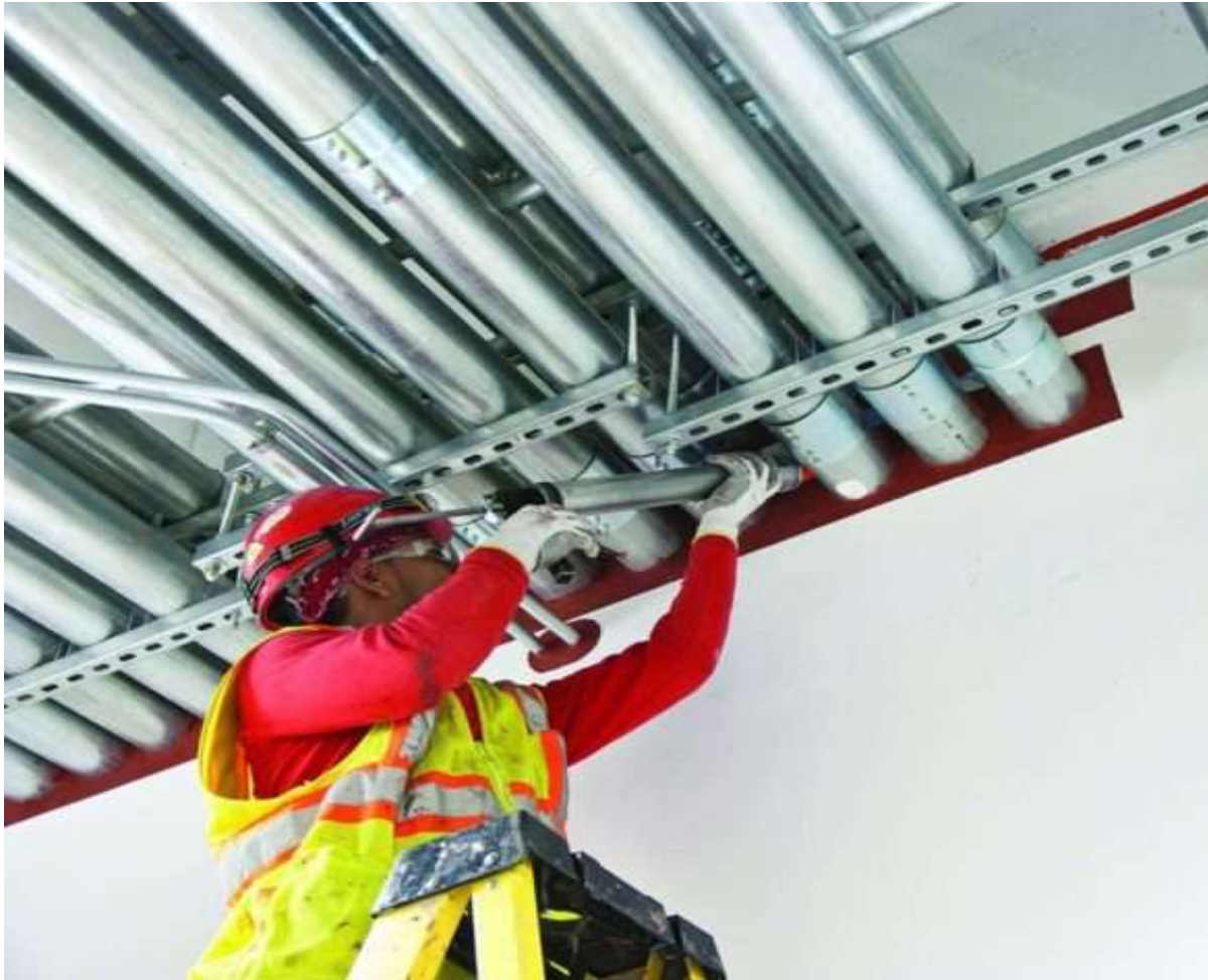
Multiple Penetration - Intumescent Sealant Application
