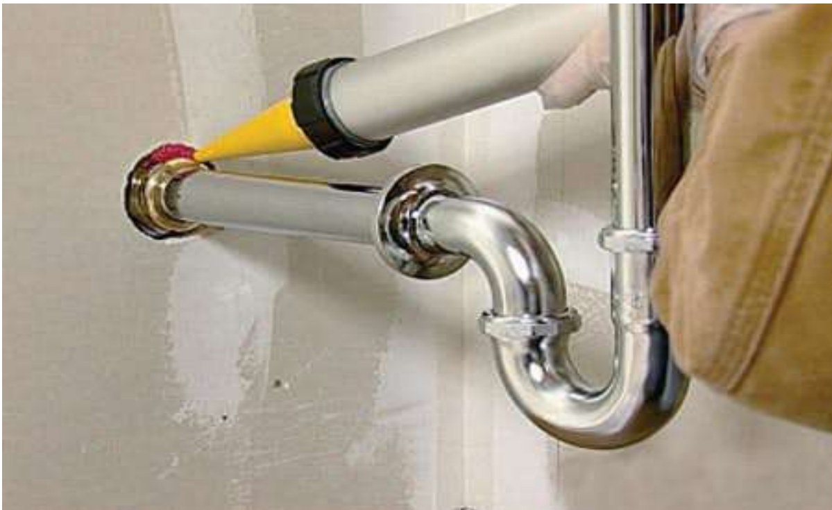
Membrane Penetration- Intumescent Sealant Application
