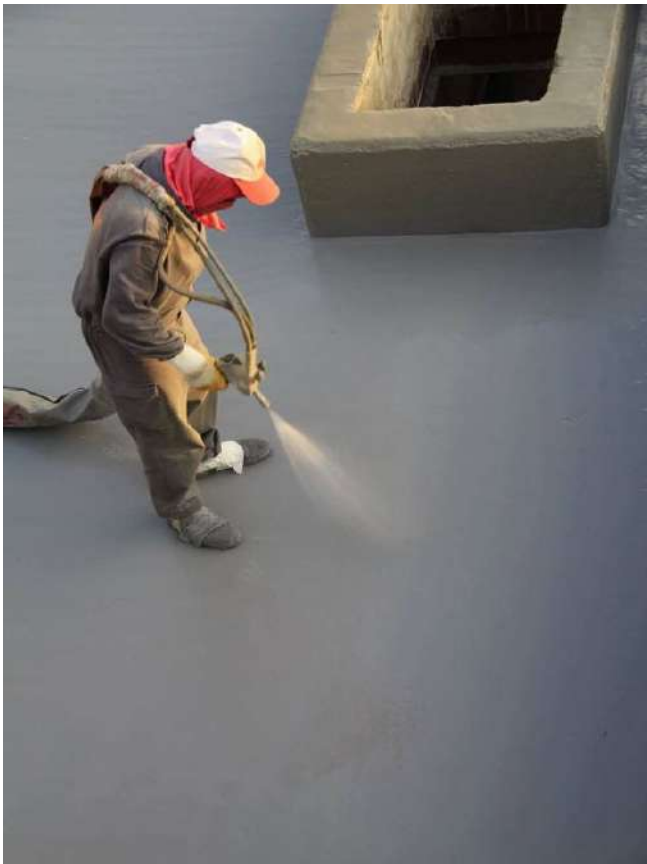
Application of Polyurea Coating
