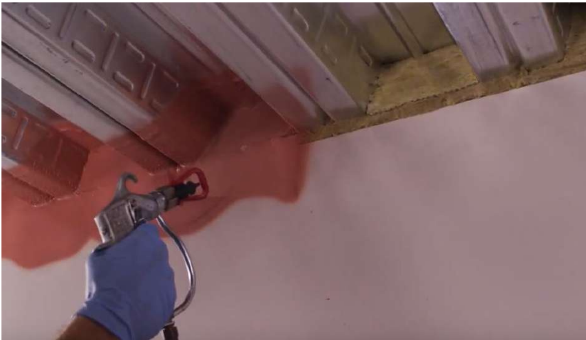
Edge Of Slab Joint Spray for Non-rated Joint System
